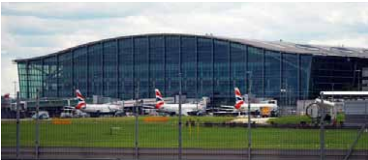
Heathrow Terminal 5 building © RGS-IBG Discovering Britain
